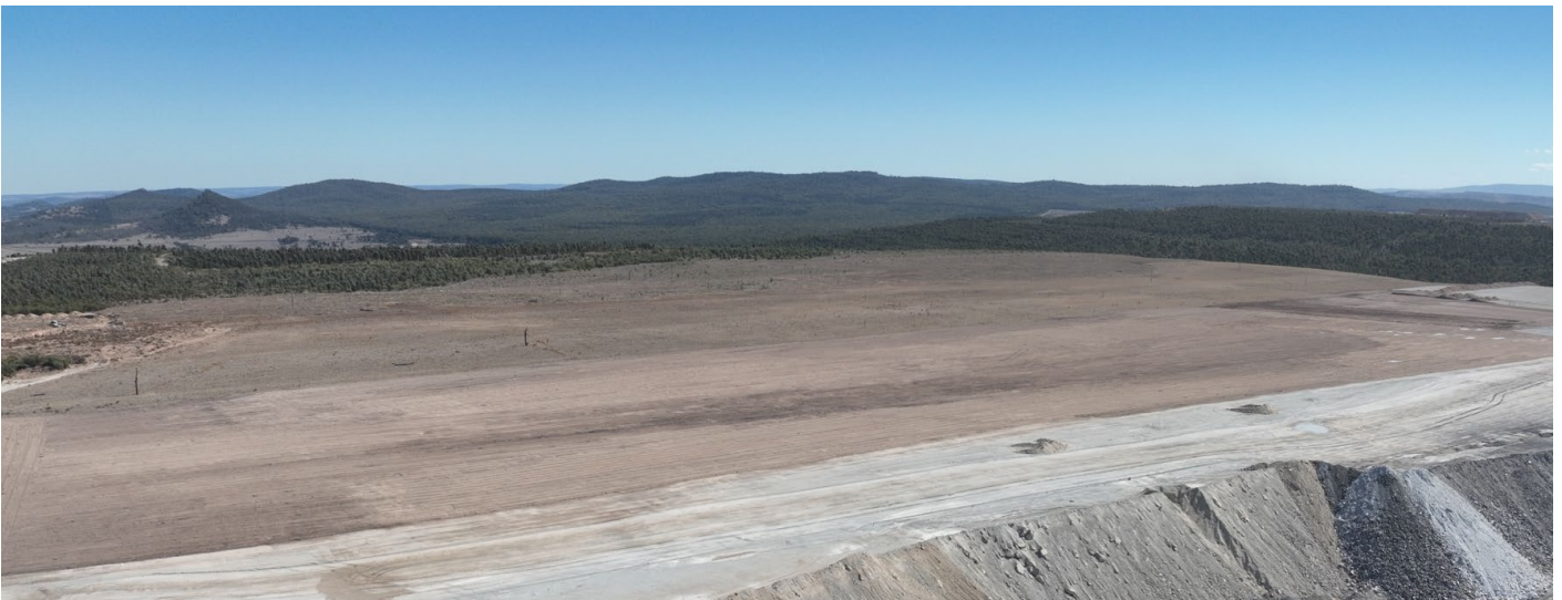
Figure 3 North Rehab – Northern Rehab Topsoil Spreading (April 2026).
