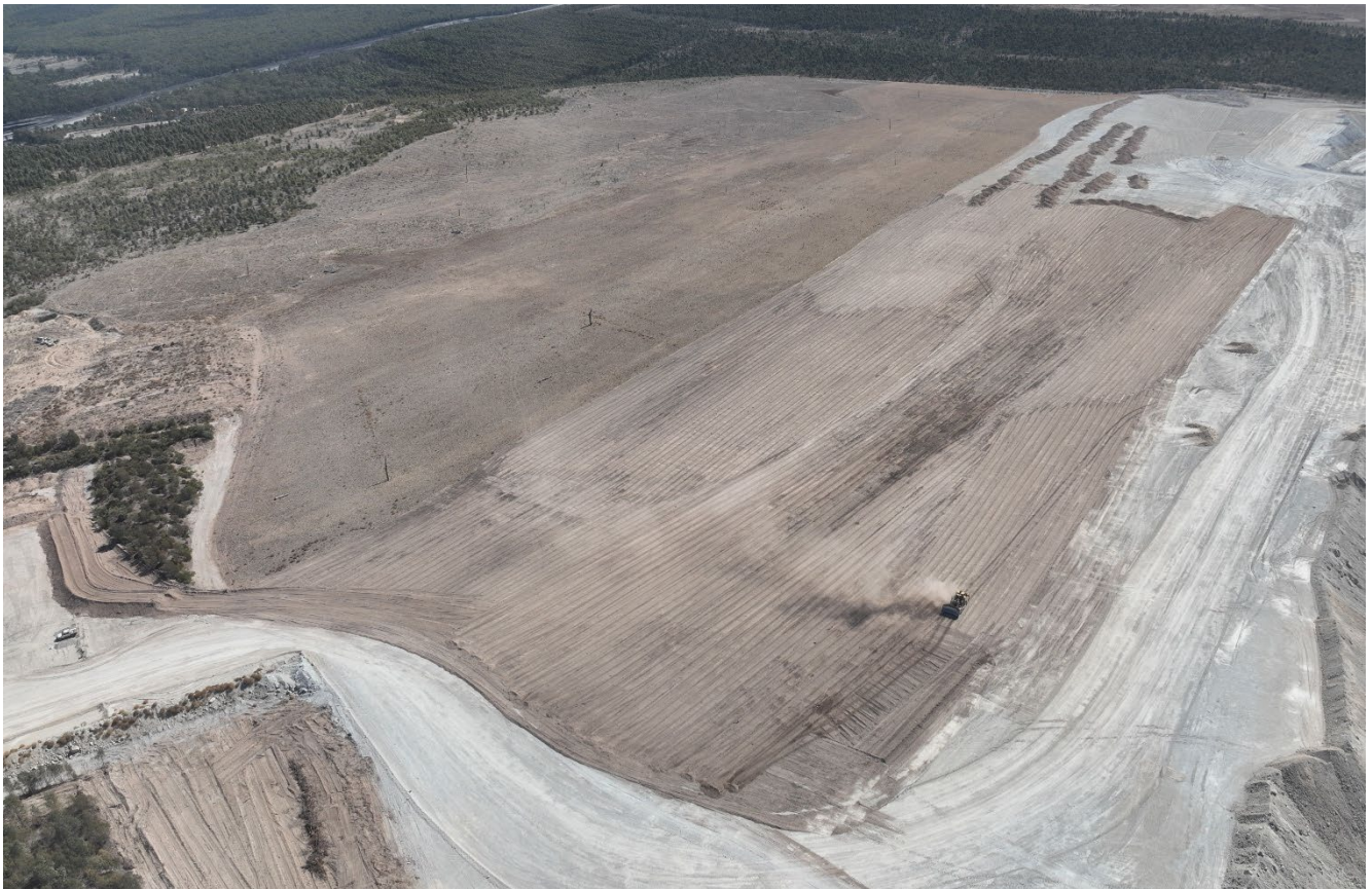
Photo taken March 2026 showing rehabilitation progression of the Northern Plateau Emplacement Rehab Area
